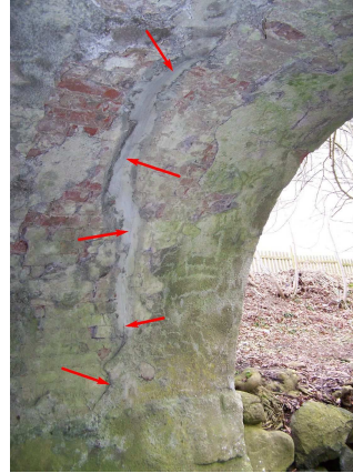
2131505_0_2009H_GEWÖLBE LINKS L-RISS
