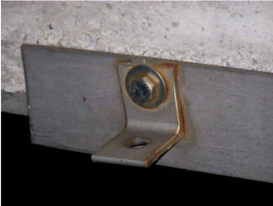
2131513_0_2009H_L-SCHLAGSCHIENE ANGEROSET
