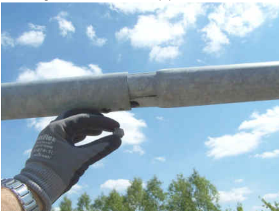
2131513_0_2009H_L-EDSP A-10 GEL-BOLZEN LOSE
