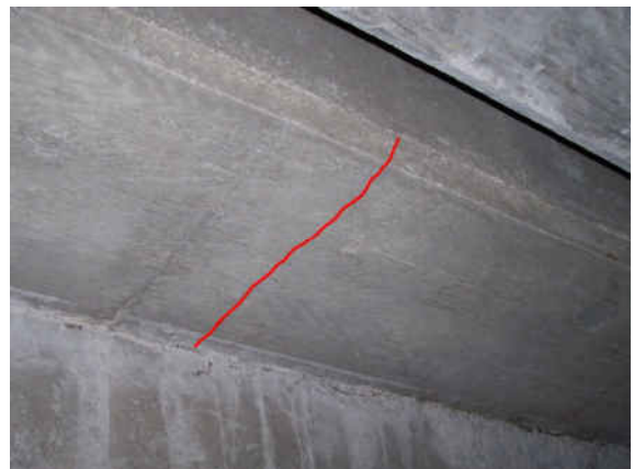
2131513_0_2009H_KONSOLE WL-V GERISSEN
