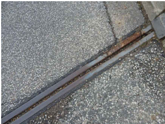
2131513_0_2022E_FÜK WL-H LINKS ANGEROSTET
