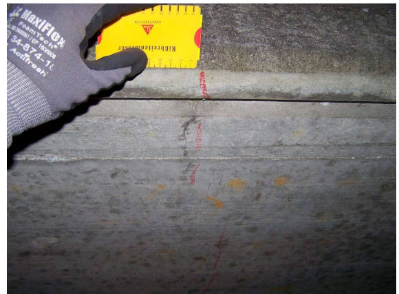
2131506_0_2009H_R-SCHUTZDACH GERISSEN
