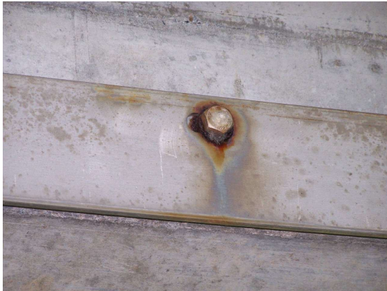
2131506_0_2009H_R-SCHLAGSCHIENE HINTEN ROSTIG
