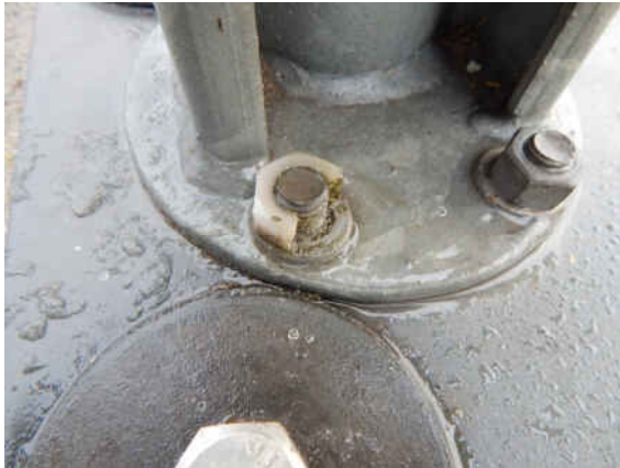
2131513_0_2025H_L-EDSP PF-8 MUTTER GEBROCHEN
