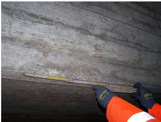
2131506_0_2009H_R-BALKEN LINKS GROBKORNSTELLE
