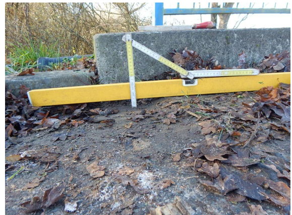
ASL_030_0_2025H_FAHRBAHN VORNE LINKS ABSACKÜNGEN
