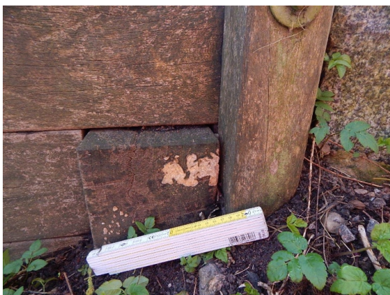
ASL_002_0_2020E_QT-1 LINKS PILZBEFALL
