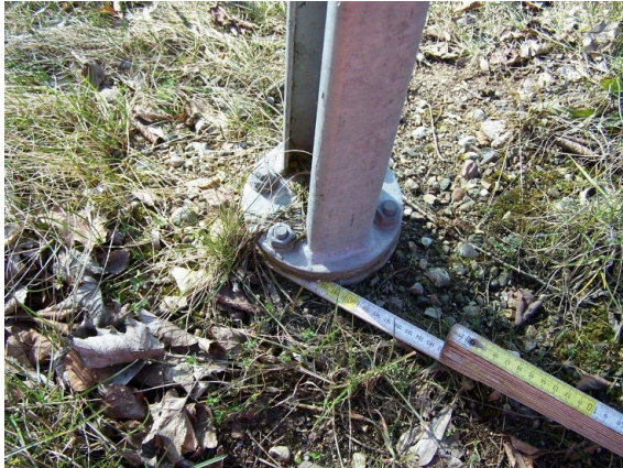
ASL_029_0_2009H_R-SPL LOSE VERANKERUNG
