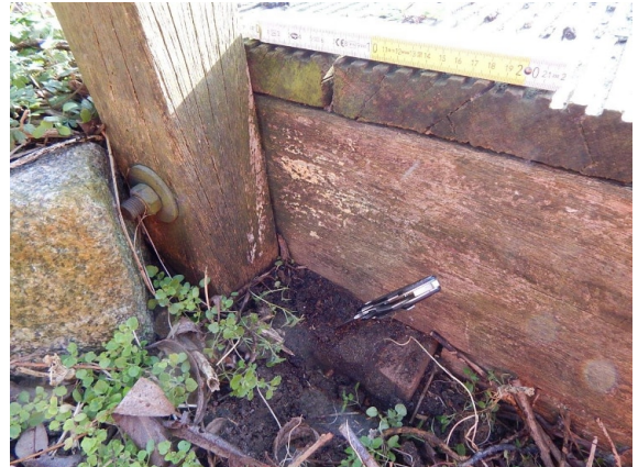
ASL_002_0_2020E_QT-6 LINKS OBEN ANGEFAULT
