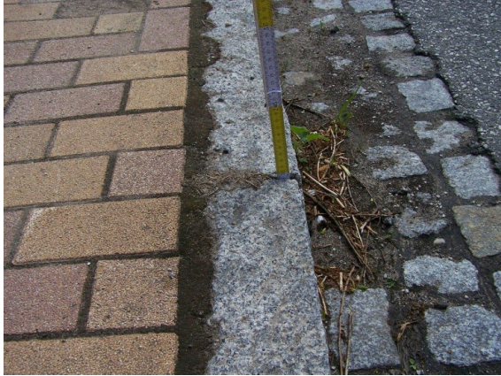
ASL_029_0_2012E_L-BORD STOSSFUGEN OFFEN
